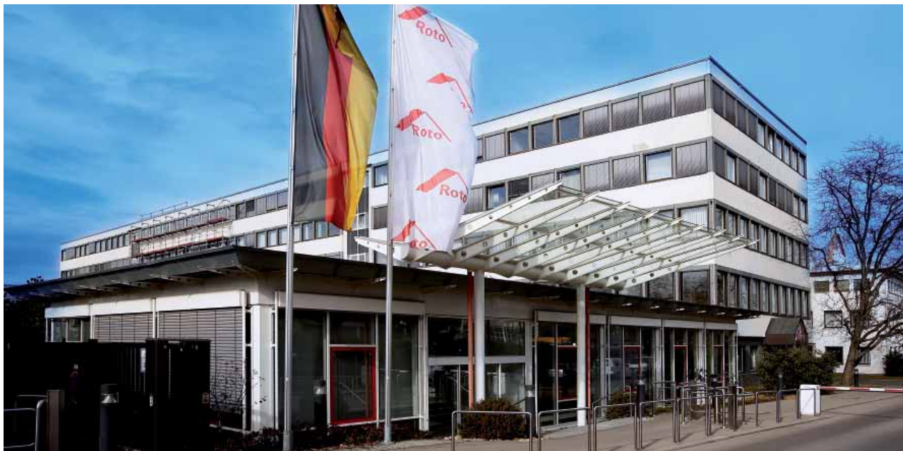
Entrance area of the Leinfelden-Echterdingen production-plant
